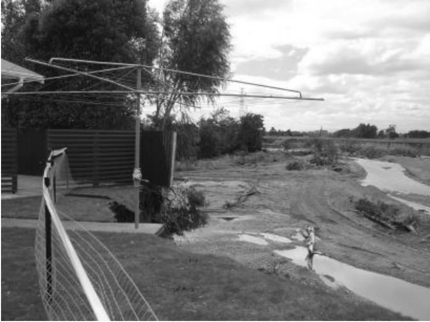
FIGURE 4.3. Flood damage from the February 2004 floods in the central North Island, New Zealand. (photo D. Johnston)
